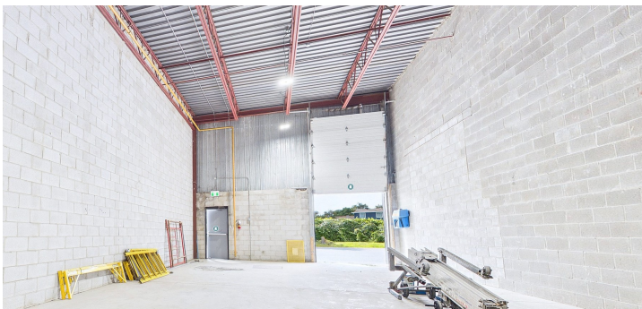
Warehouse, clear height and loading door
